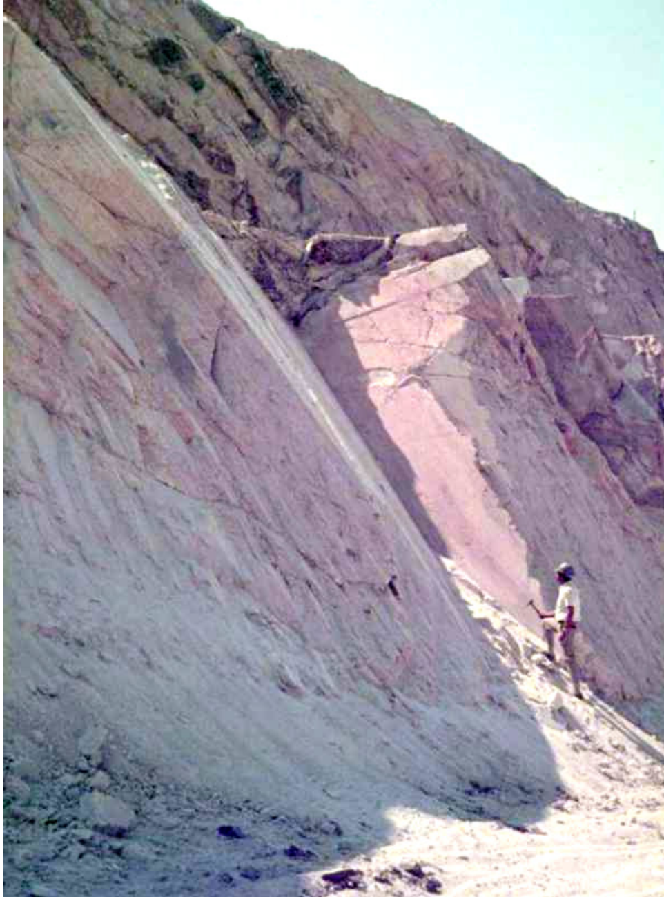
Figure 4: A wedge failure controlled by intersecting structural features in the rock mass forming the bench of an open pit mine.
