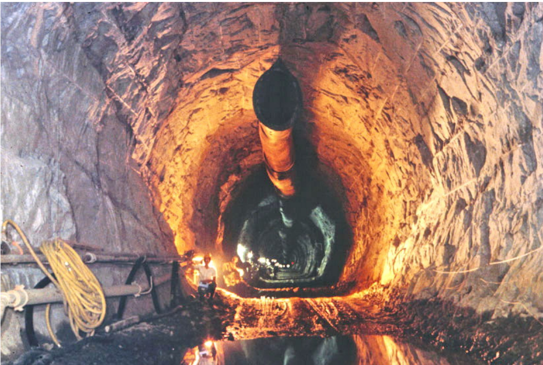
Figure 1.11: An example of good blasting in a tunnel.
