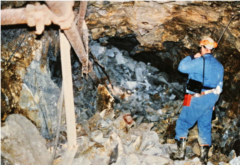
Figure 3: The results of a rockburst in an underground mine in brittle rock subjected to very high stresses.
